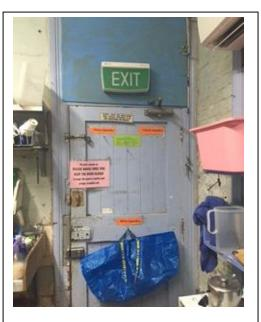
**Photo 1:** Exit Light not Illuminated. No door lever for exiting building. Door also swings against direction of egress.
