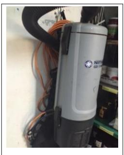
**Photo 2:** No electrical testing and tagging or portable electrical equipment
